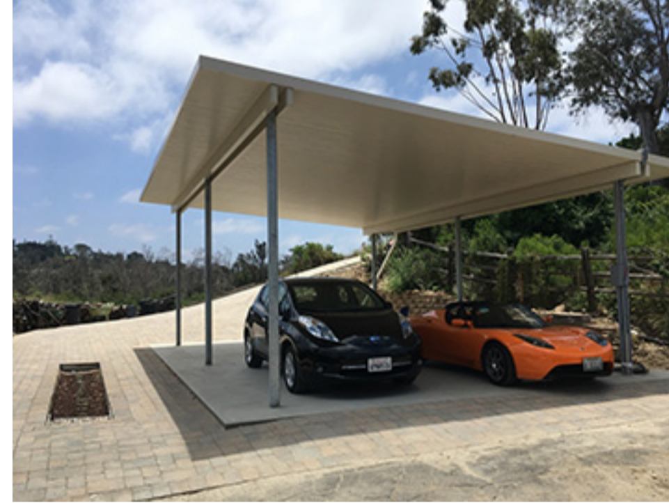
Solar Carport also provides Shade
