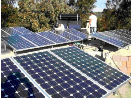
Phase 1 being installed on rooftop, 2003. These make about 60% of our solar.
