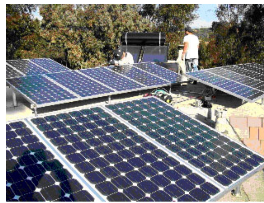
Solar PV panels being installed. 2003
